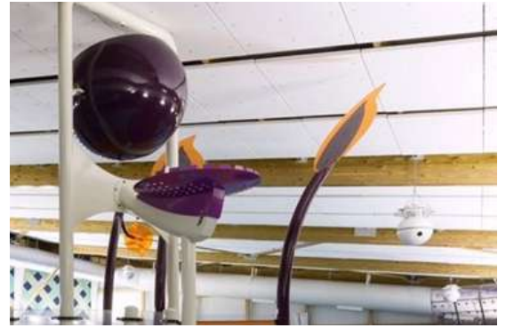
b. Quietspace® Panels with gaps to keep the roof cavity well-ventilated
